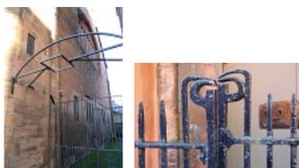
The double doors have broad strap hinges which meet in the middle, resembling a continuous band, with only a slight peak to mark where the two leaves
