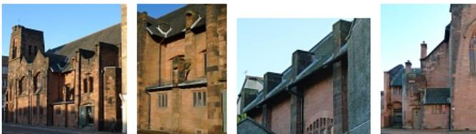
All these disparate parts are pulled together by the square tower at the corner of Springbank Street. It tapers for the upper third of its height and has a polygonal stair turret embedded in its W. face. These features, and the clasp buttresses at its base, are derived from the medieval tower of All Saints church at Merriott, Somerset, which Mackintosh had sketched on a visit in 1895.<sup>11</sup>
