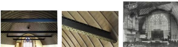
The chancel has an open roof of unusually elaborate construction, despite being largely hidden by the chancel arch. Its purlins are carried on shallow arched braces with square pendant ornaments, resting on corbels. Where the rafters meet the wall, they are gripped by pairs of timber brackets, a variation on the treatment of the roof of the central hall at Martyrs Public School.
