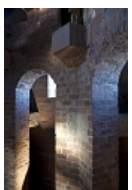
Brick construction inside tower
