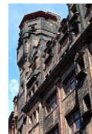
Tower from below
