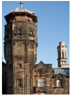
Tower and chimney
