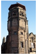
Tower from N.W.
