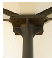
Cast-iron capital, top floor
