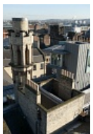
Chimney top and roof of main stair
