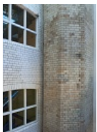
Chimney shaft and windows to stair
