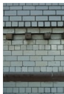
Glazed brick on E. elevation of Mitchell Street building
