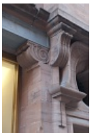
Corbel and cast-iron lintel, Mitchell Street
