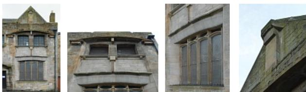
At the opposite end of the front, a D-plan, tower-like projection contains the stairs, a feature that Mackintosh would soon use again at Windyhill and The Hill House. The lower windows follow the slope of the stairs; those at the top have a slight notch in the lintel, giving them the merest hint of an ogee head, and pairs of curious bracket-like projections above.
