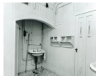
Oak Room, basement lavatories, 1971, photograph by Eric Thorburn
