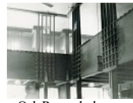
Oak Room, balcony balustrade, 1940s, photograph by Thomas Howarth
