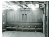
Basement billiard room 2, S. wall, 1970
