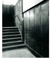
Basement stairs, 1971, photograph by Eric Thorburn
