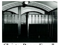
Cloister Room, E. wall, 1950
