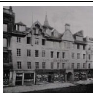
Exterior, Argyle Street, Builders' Journal and Architectural Review, 15 April 1903, p. 131
