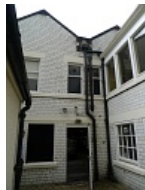
N. elevation of internal courtyard
